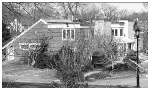
Snow Library “looks like a nice building,” said Kevin Galligan, but staff are “overcoming challenges every single day.” ED MARONEY PHOTO
